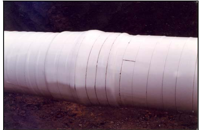
600 Series Coating applied on a rehabilitation project.
