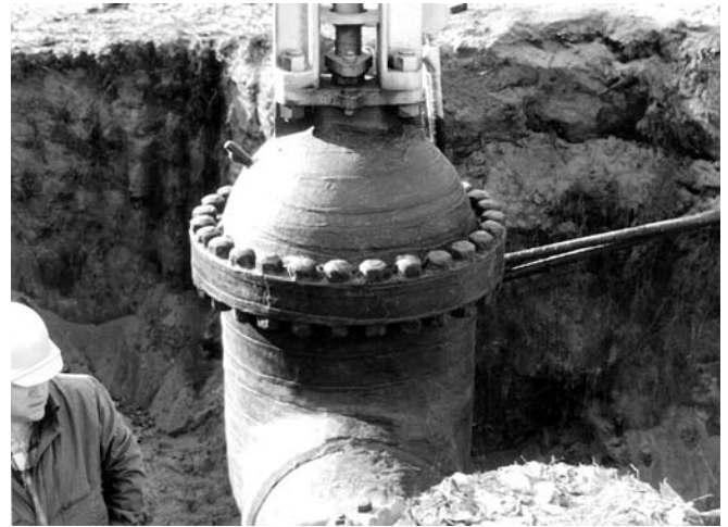
#1 Wax-Tape can be applied to small and large valves, flanges and bolts.
