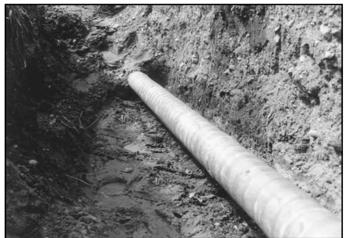
Section of 16" pipe reconditioned using #1 Wax-Tape and Glas-Wrap.
