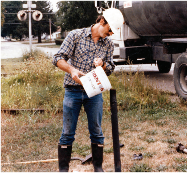
Pre-Con® being poured into the casing through the casing vent.
