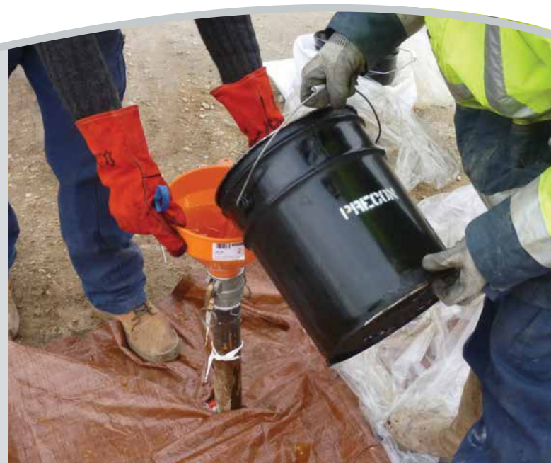
Trenton Pre-Con® mitigates any corrosion that would be caused by water left in the casing.
