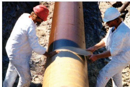
Finished application of Innercoat® wax is overwrapped with Guard-Wrap™ wrapper.
