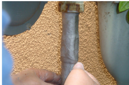
8. Press the pad of Wax-Tape® wrap firmly to the pipe. Press to eliminate any bubbles and smooth the lap seams and end seams to ensure that they are sealed.
