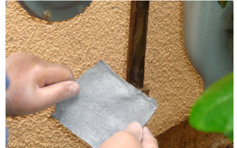
6. Wipe hands clean of primer. Remove pad of Trenton Wax-Tape® wrap from package and remove the backing paper.
