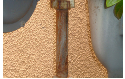
3. Wipe the area clean. Surface should be wiped as dry as possible.
