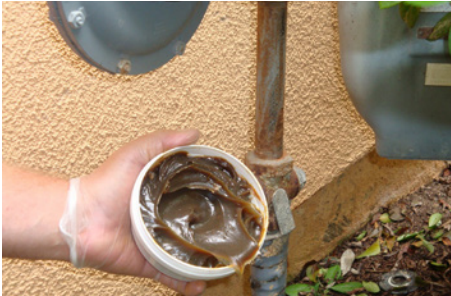
4. Hand apply the primer. Firmly rub and press the primer onto the surface to displace the moisture and ensure that the primer is adhering to the metal surface.
