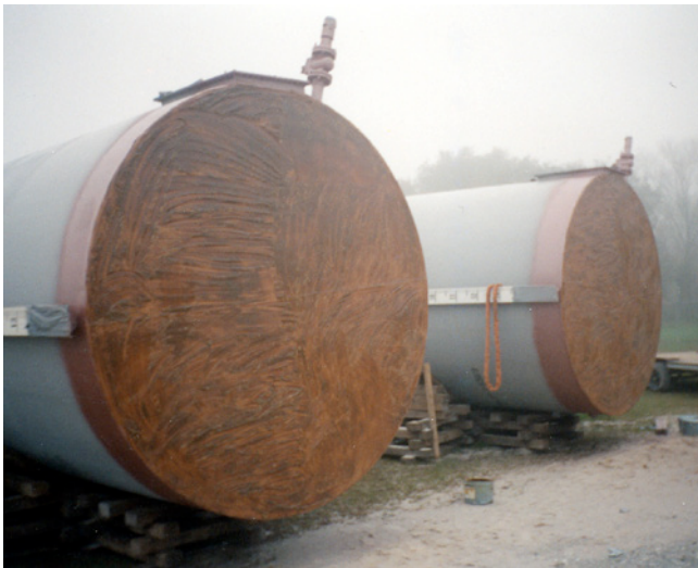
Temcoat applied to pipe surface. It will then be wrapped with Poly-Ply™, Guard-Wrap™ or Wax-Tape®.
