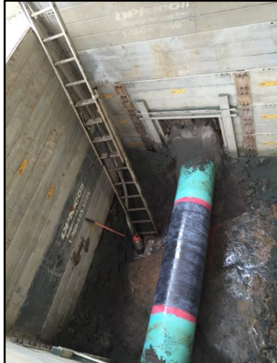
BlackDiamond® repair successfully installed and cured
