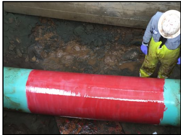
Application of epoxy primer for corrosion protection and enhanced adhesion
