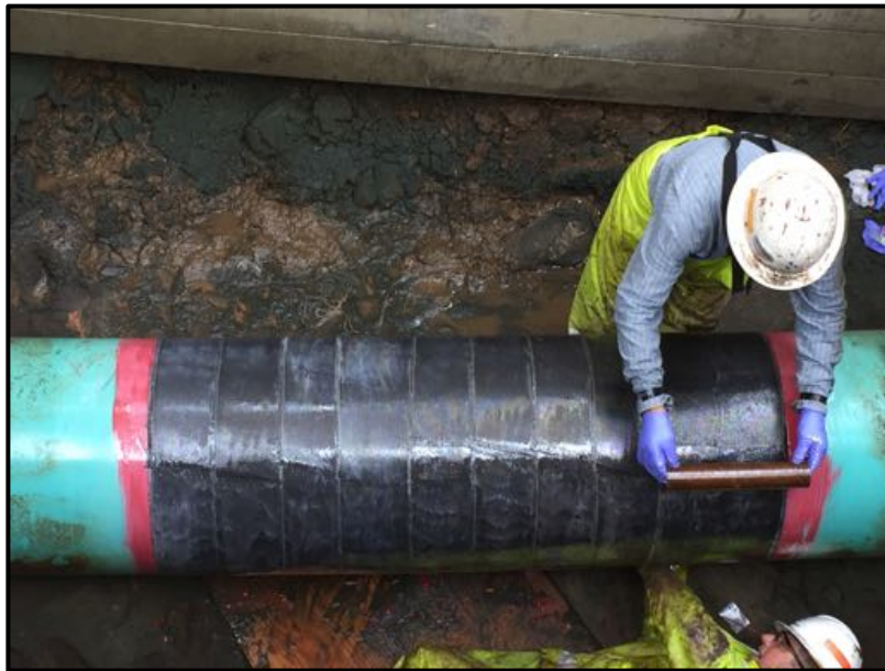
Application of carbon fiber saturated with epoxy wet out
