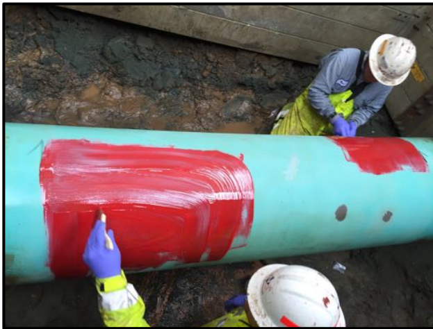
Application of epoxy primer for corrosion protection and enhanced adhesion
