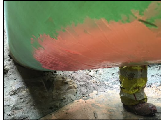
High compressive modulus load transfer epoxy used to smooth anomaly
