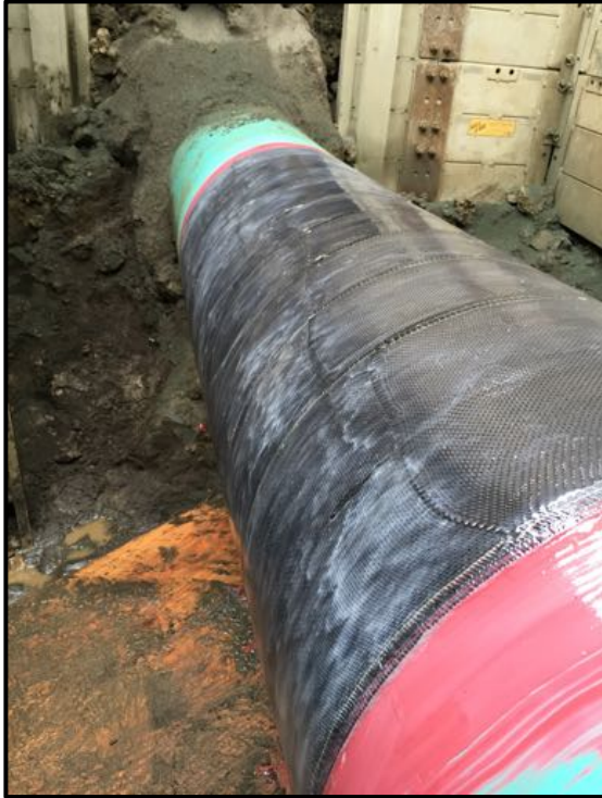
BlackDiamond® repair successfully installed and cured
