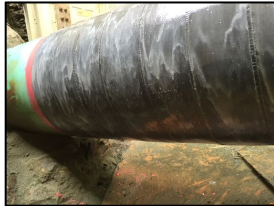
Before and after of repaired dented area
