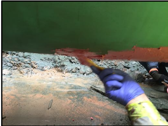
High compressive modulus load transfer epoxy used to smooth anomaly
