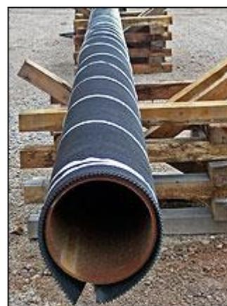
RockGuard can be installed along the pipe or around the pipe as per the diagrams below, and can be secured by means of polyester strapping tape.
